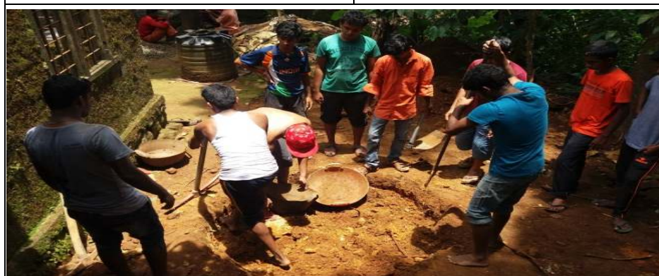
Construction Of Toilets For Tribes In Peringassery
